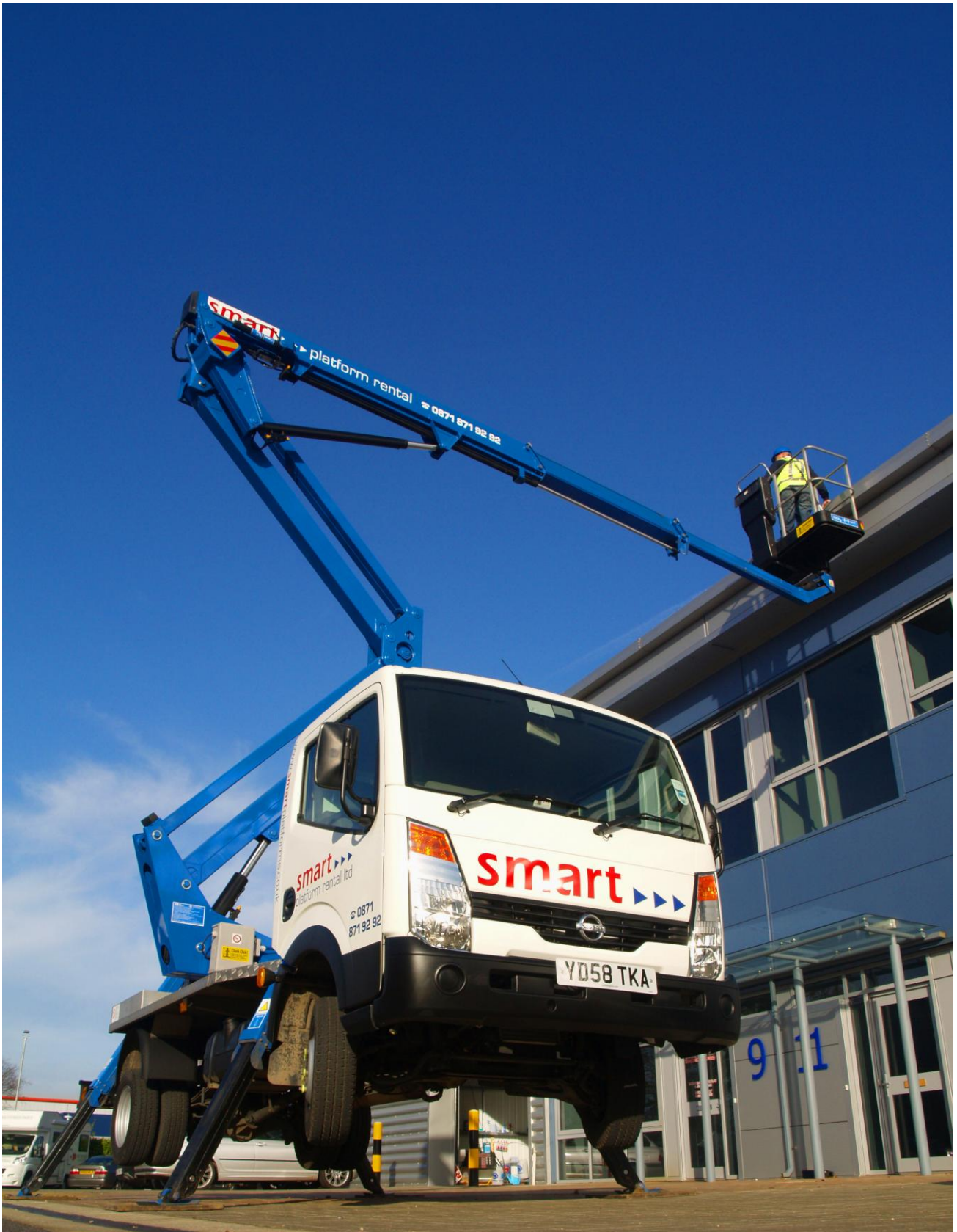
A new Z19 working near the new Hemel offices
